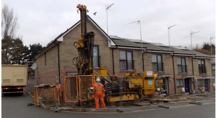
This was an Emergency Investigation and Treatment Works Contract which was undertaken following the formation of a ground collapse directly outside a property on this newly constructed housing development in Plumstead, South East London. The residents adjacent to the collapse were immediately evacuated and the initial collapse filled with concrete. Peter Brett Associates were appointed by the client to design and supervise a site investigation followed by a ground treatment scheme.
